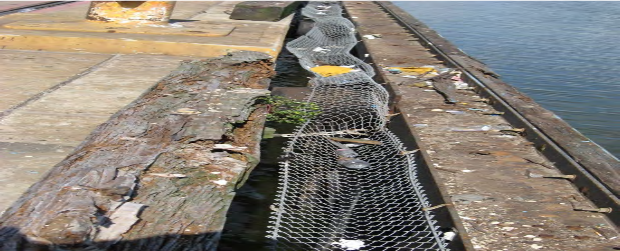
This is an annual fender system maintenance at Barbours Cut and Bayport Terminals, mainly the replacement of safety net and nuts and bolts.
